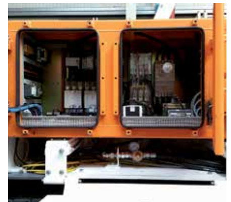
Inside view switch gear cabinet
